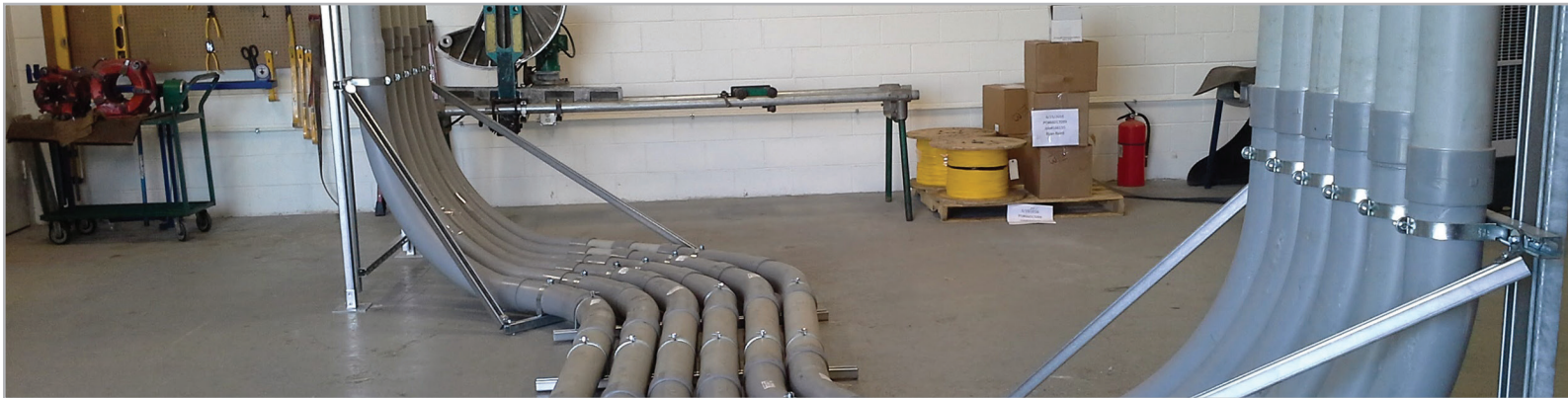
CONRAC Duct Bank for ATS Extension
