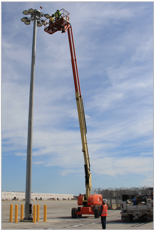
Crews 60' in the air, installing high-mast lighting at O'Hare International Airport.
